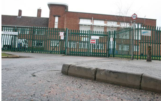
Large curb protruding out at the entrance to the school which causes problems for delivery vehicles
