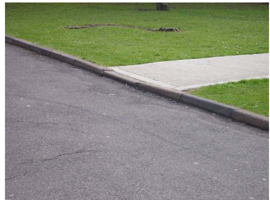
Drop curbs at pedestrian entrances – these have now been removed
