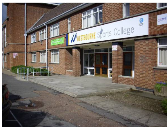
Before (patchy/uneven surface and curb)
